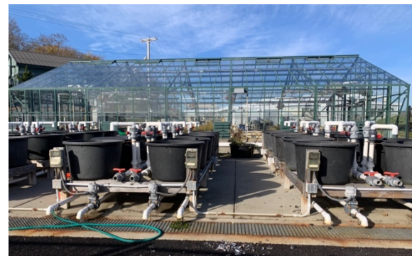
The Marine Science Center Tank Farm.
